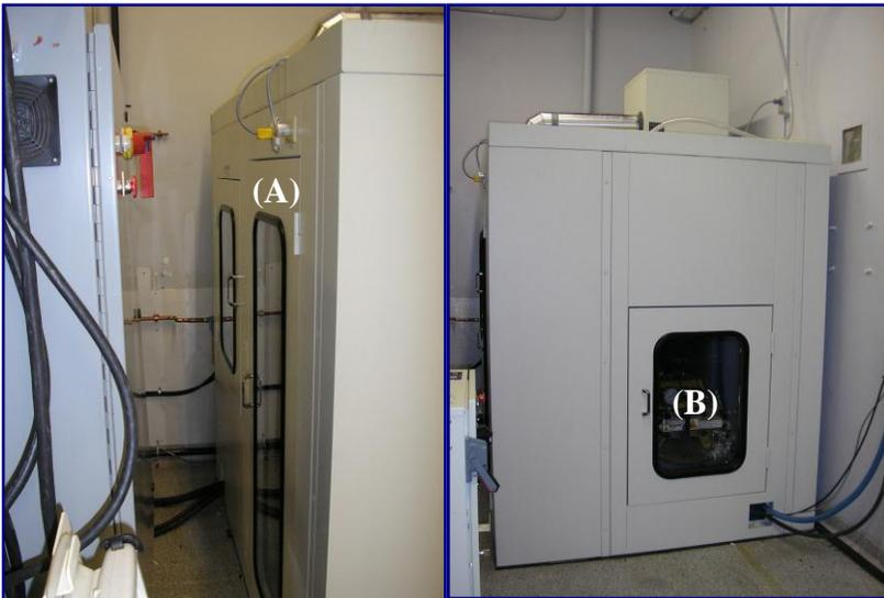
Fig. 9. Close-up views of the pump enclosure. (A) Access door for VFD and control box, (B) Access door for accumulator and other accessories.
